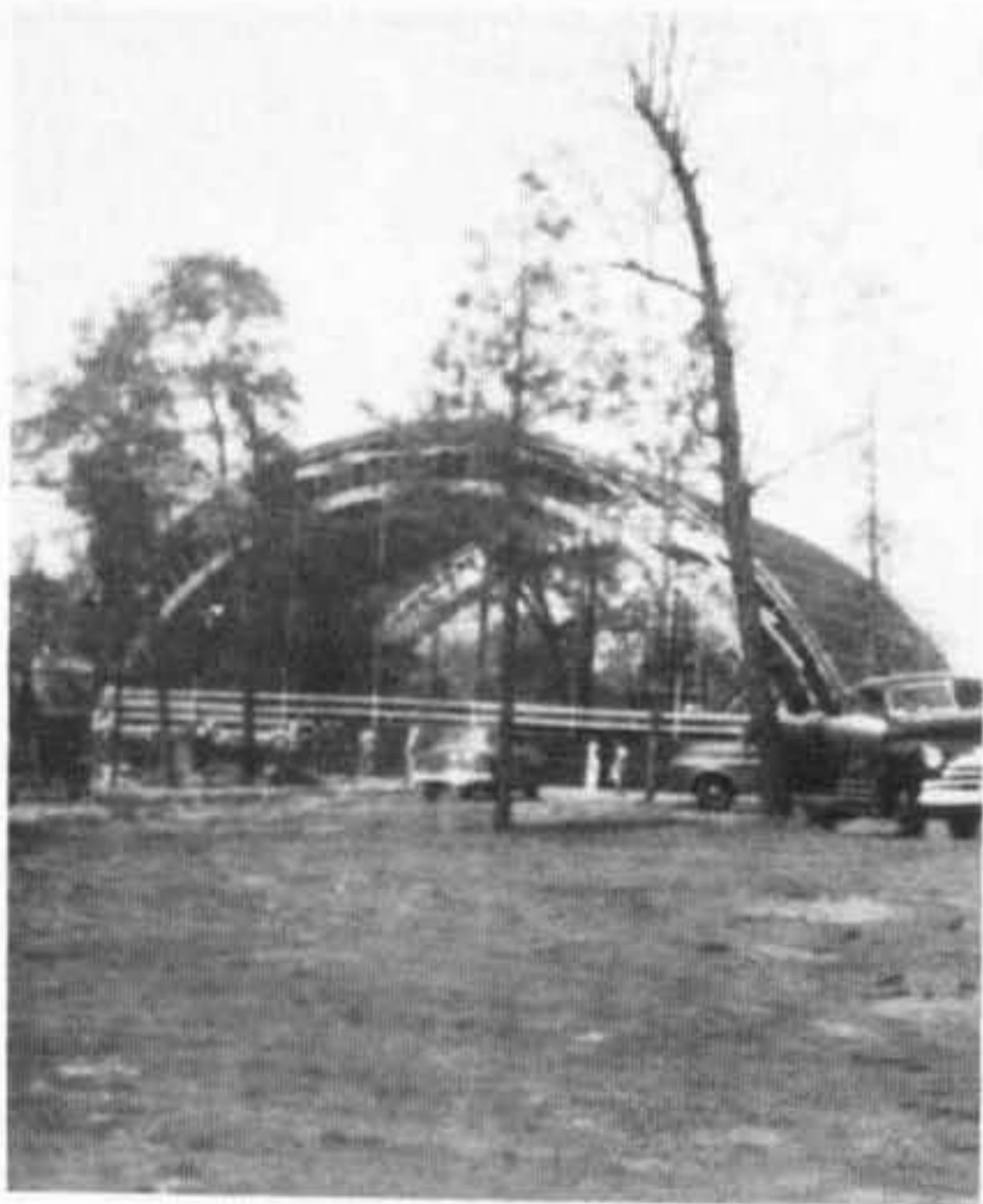
Just enough, completed to meet the first year
